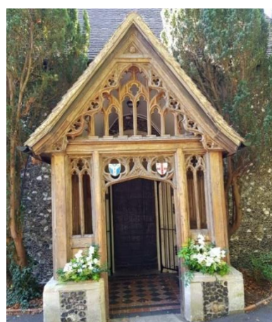
Ledges on North porch
